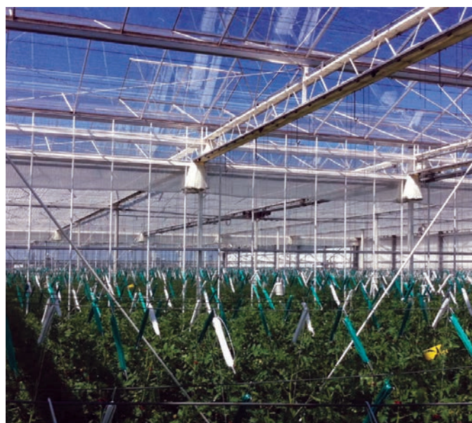
Situation A: no shading in the front of the greenhouse versus situation B: shading with high grade light diffusing HARMONY climate screen greenhouse at the back.
